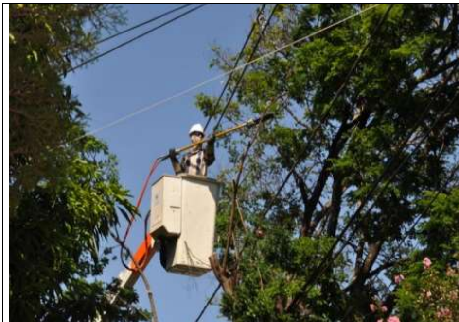
Figure 4: Worker performing vegetation pruning activity.
