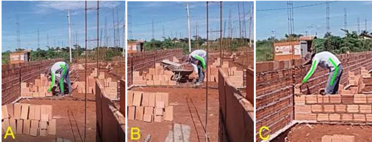
Figure 3 – Execution of Masonry Elevation (Initial Rows)
